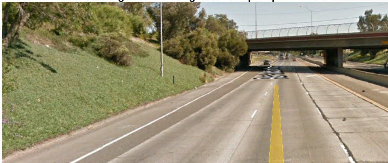
Figure 2: Below grade with up-slope
