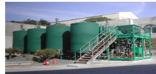
Brown Grease Processing System at San Francisco's Oceanside Wastewater Treatment Plant (Source: SFPUC)
