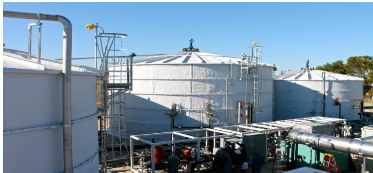
Brown Grease Processing System at San Francisco's Oceanside Wastewater Treatment Plant (Source: SFPUC)
