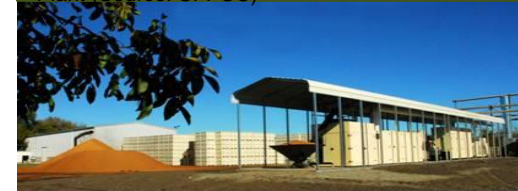
Community Power Corporation's BioMax 50 demonstrated in Winters, CA for almond shells (Source: CPC)
