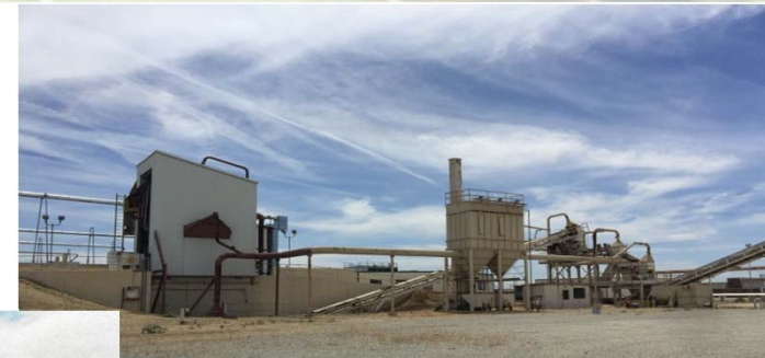
Feedstock Unloading, Handling & Processing
