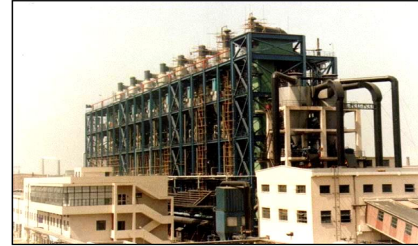
800 ton per day U-GAS® coal gasification plant in Shanghai, China
