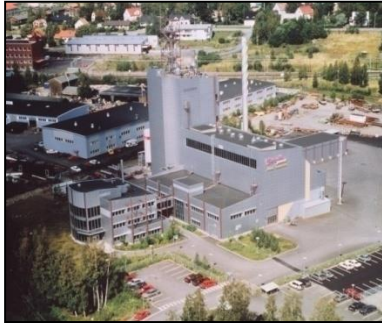
80 ton per day Gasification Pilot Plant in Finland using biomass & coal
