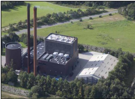
165 ton per day CHP Plant in Skive, Denmark using wood
