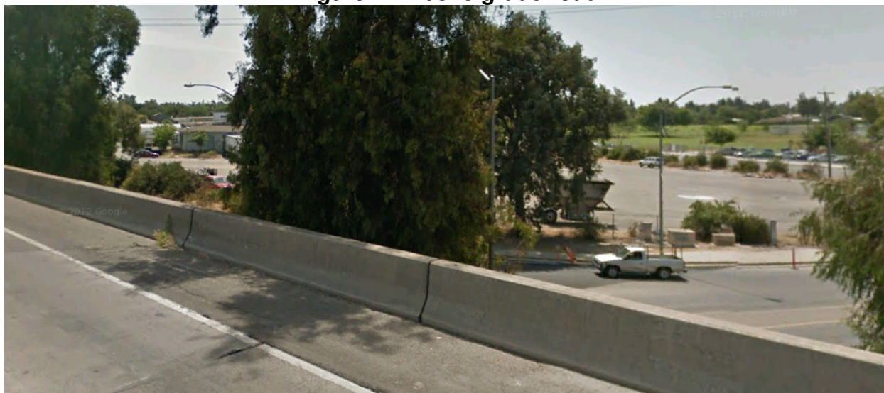
Figure 1: Above grade road
