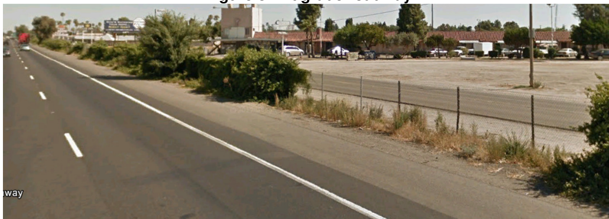
Figure 3: At grade roadway
