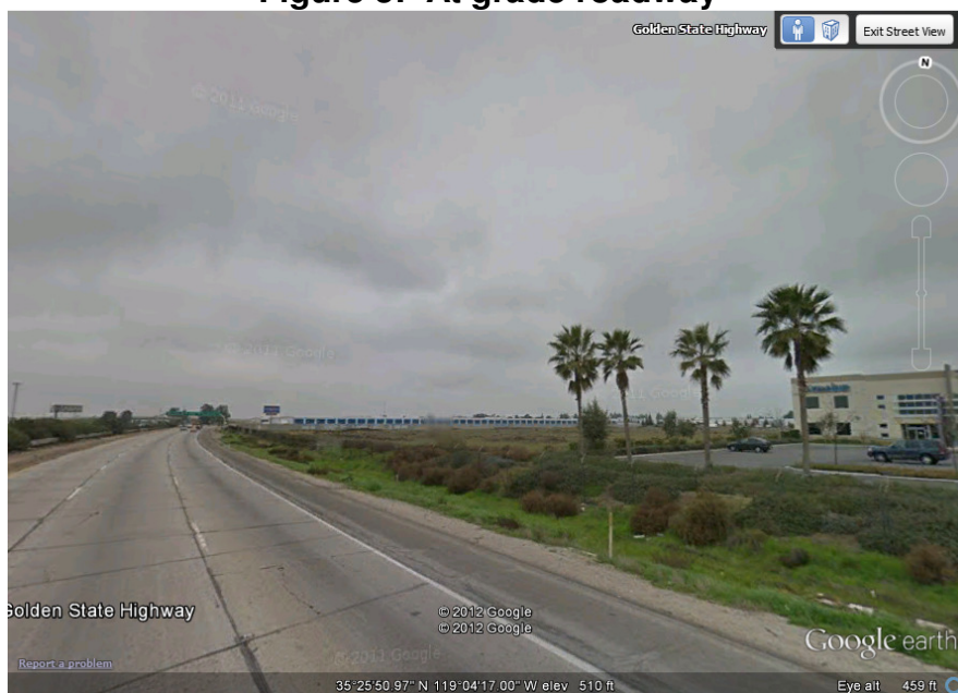
Figure 3: At grade roadway
